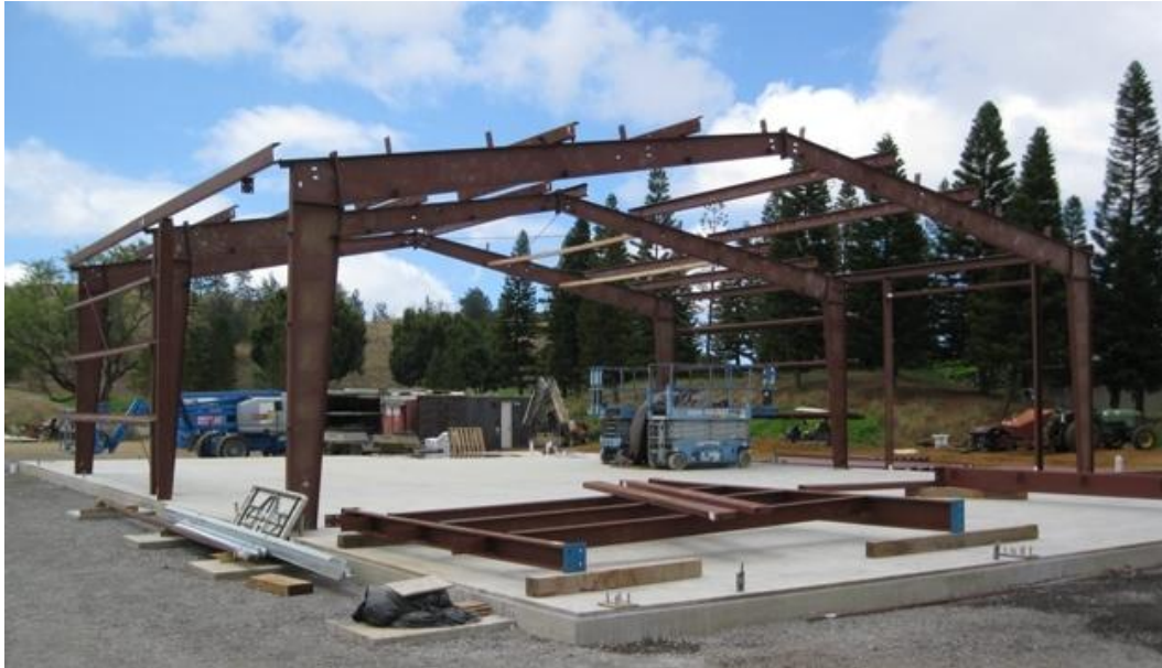
New maintenance and storage building under construction.
